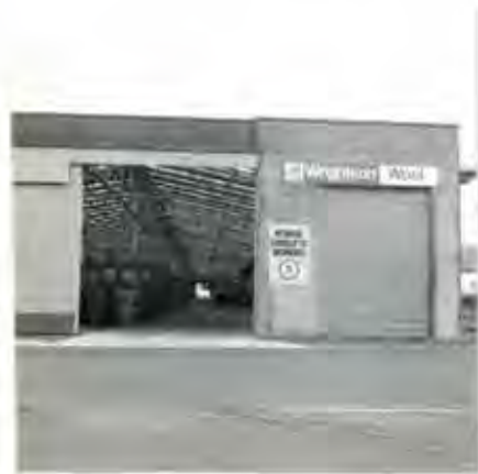
Wrightson wool storage facility on Strathallan Street, Dunedin.
