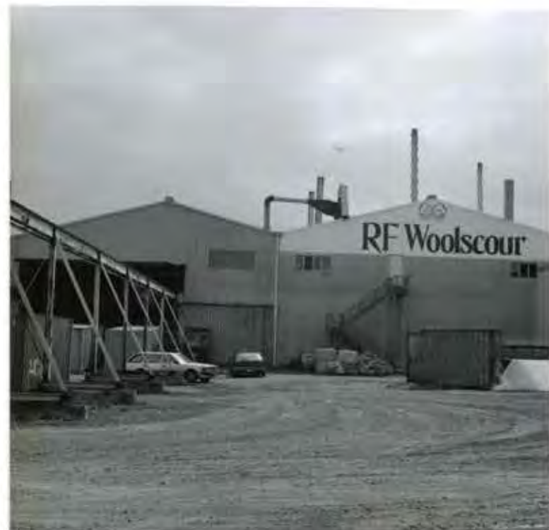
RF Woollscour at Parry Street. The plant operates around the clock.
